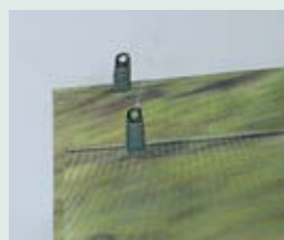
Glued-in metal rod with metal clip
